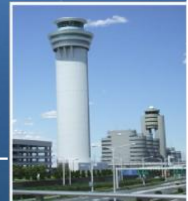
【Reference】 Start operation of new control tower (12 th January 2010)
